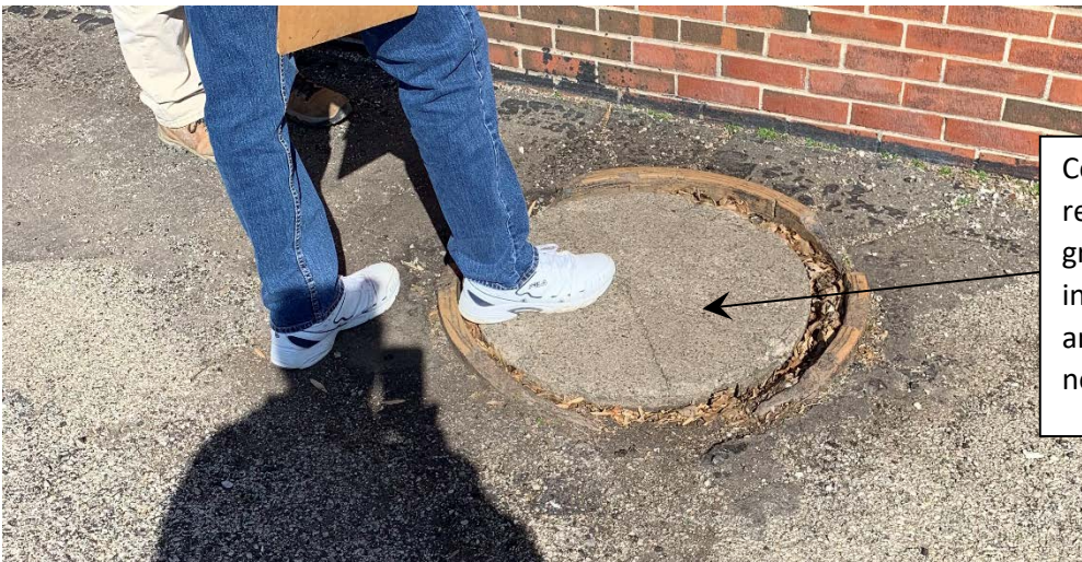
Photo C – grease interceptor lid
